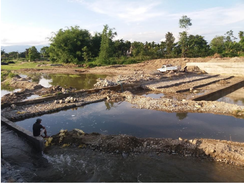
Headworks Site of Hadiya Regulator ISP under CMIASP-AF
