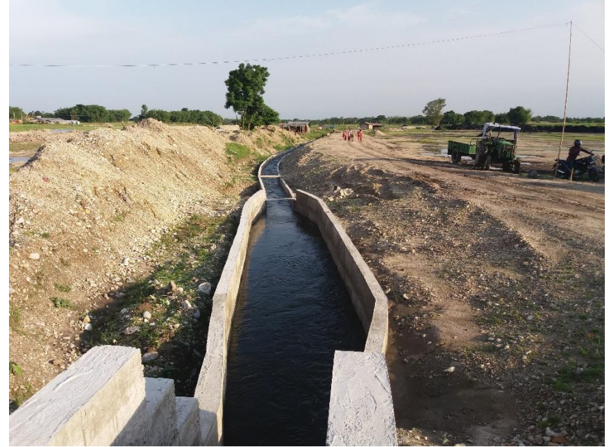
Main Canal with desilting basin of Hadiya Regulator ISP
